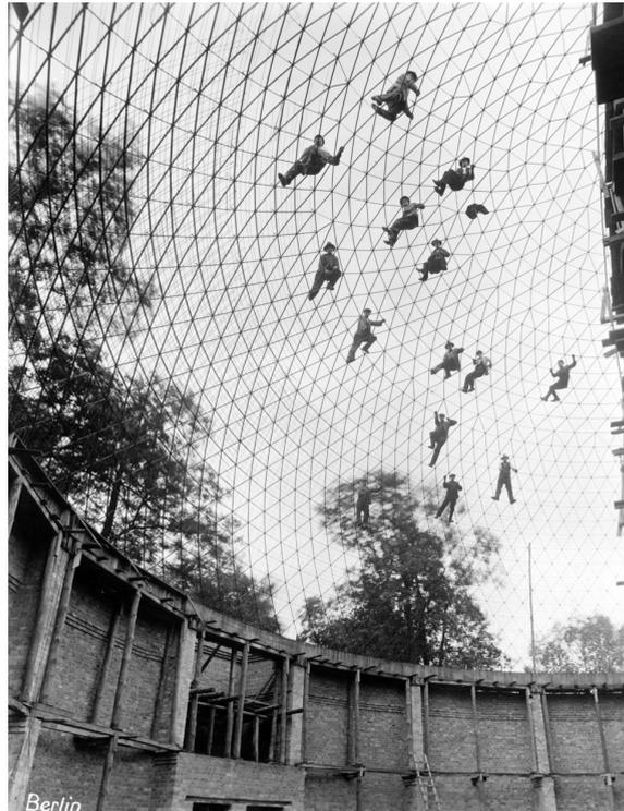
Fig. 2: Construction workers cling to the steel network of the Berlin planetarium under construction, early 1927. Courtesy Carl Zeiss Company Archives.
