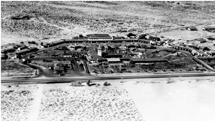
Source: Historic Aerial Photograph
