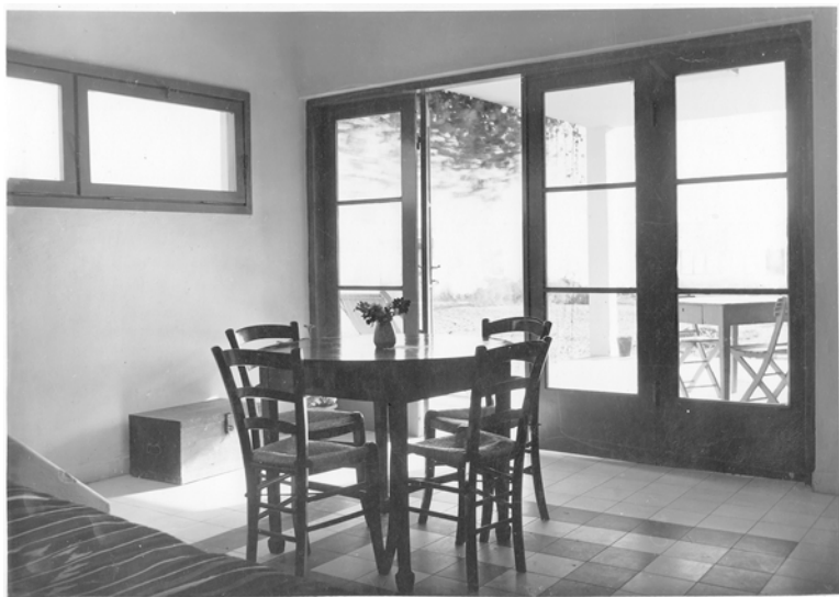
Figure 3: Interior, Goldschmidt House, Tel Aviv, 1931. Source: Courtesy of the Goldschmidt family, Ramat HaSharon, Israel.
