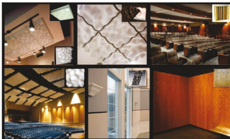
Figure 17. Top row left to right: 2D Omniffusor and Skyline layin T-bar ceiling treatment; 2D Harmonics T-bar layin ceiling treatment; Oriented 1D Modffusor wall treatment. Bottom row left to right: 2D Bicubic ceiling clouds; Stretch fabric covered 2D BAD panels; Exposed wooden furniture grade BAD panels.
