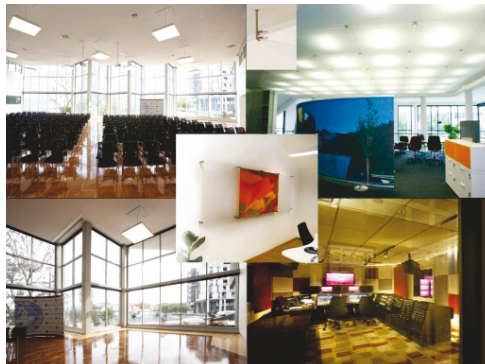
Figure 12. Top left: transparent foil window treatment; Top right: translucent foil radiant ceiling treatment; Bottom left: transparent microslit panel window treatment; Bottom right: transparent microslit panel window treatment; Center: digitally printed microslit panel.
