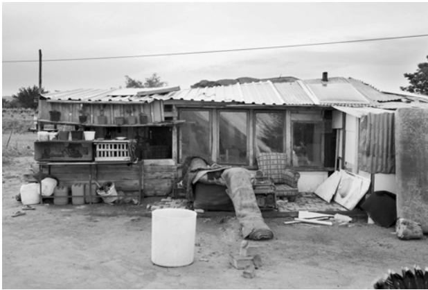
Figure 7.9: Makeshift vineyard shed in Ürgüp
