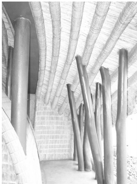
Image 2.2: ‘Inner rings’ of the roof of the main building of the Royal Kasubi Tombs, reeds tied with sisal rope.
