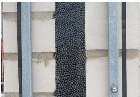
Polystyrol (EPS) in der Hohlschicht
