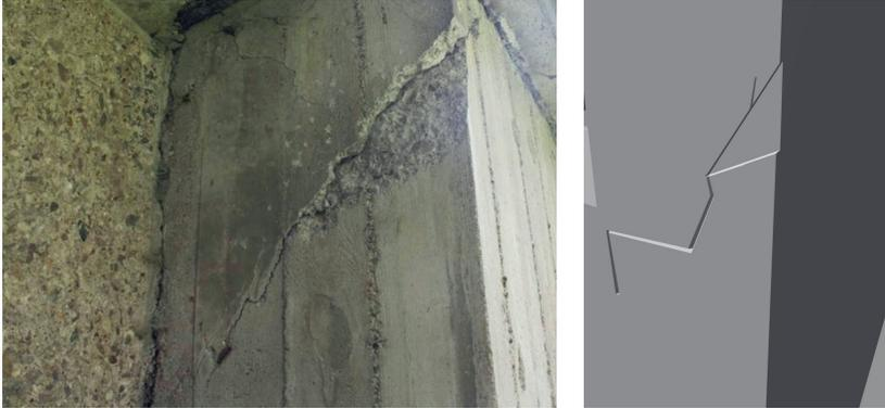
Figure 5.12: Representation of a spalling at the abutment.
