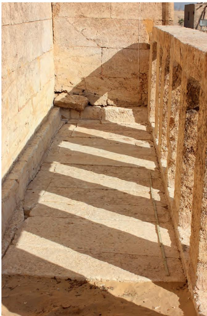
Fig. 5: Preserved pavement between naos and balustrade; 2015
