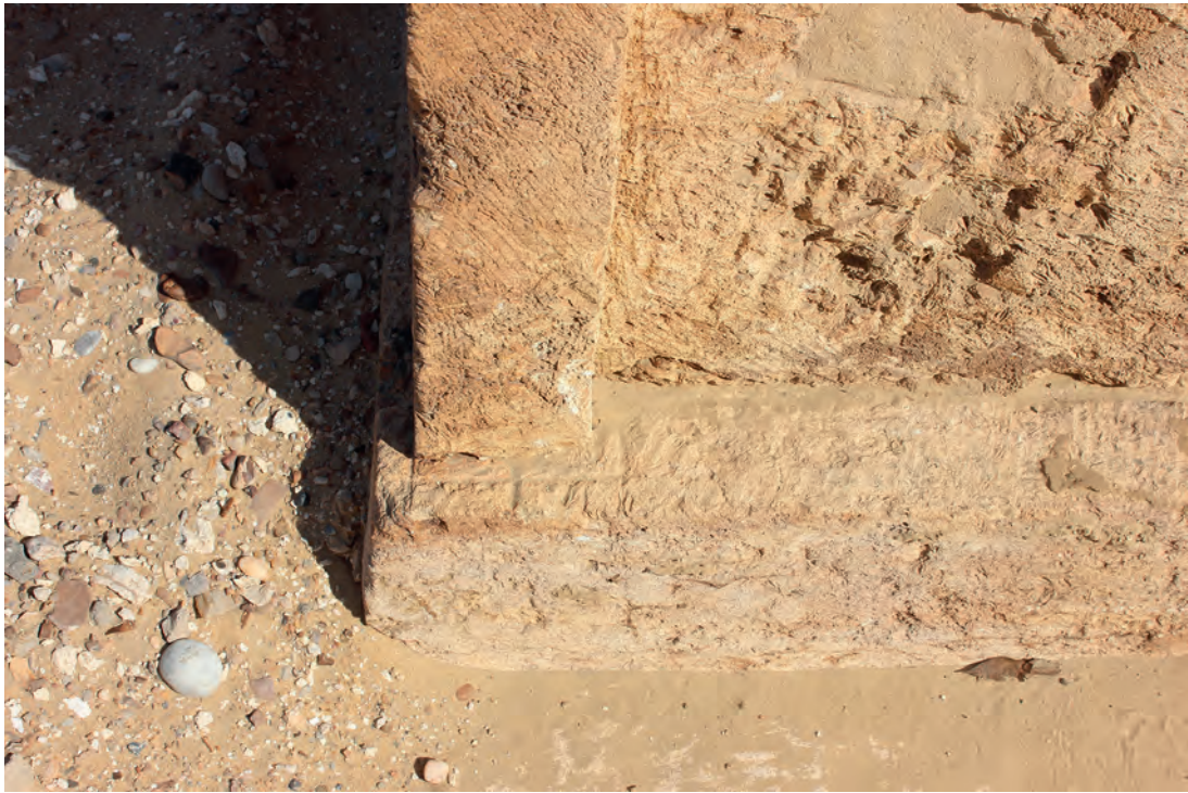
Fig. 6: Incision on top of the euthynteria indicating the future position of the round bar of the southwestern corner of the naos; 2015
